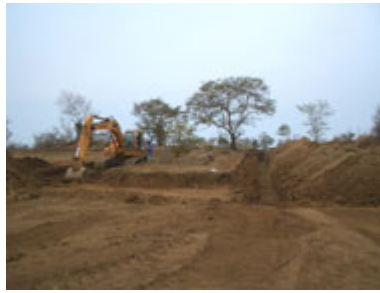
Machinery working at future avenue
