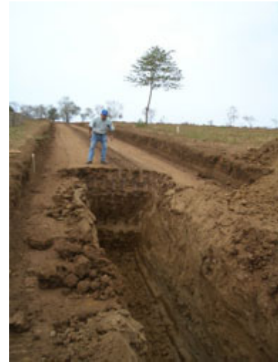
Trench for potable water system
